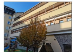
MI – Via Bordoni 2 Office and Kindergarten NRA: 2.500 sqm
